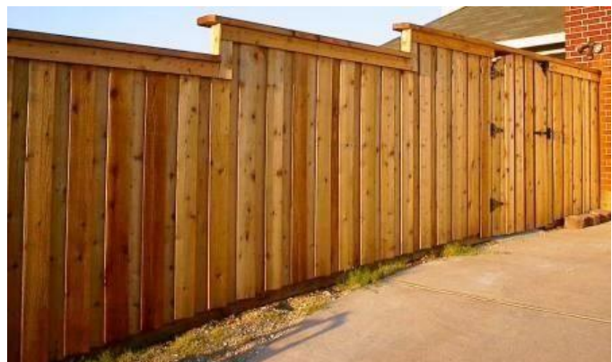
Stepped board on board or shadowbox
