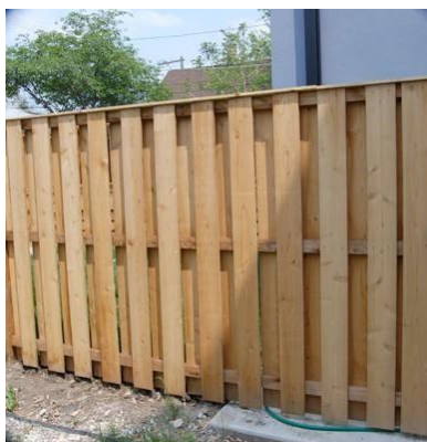
Board on board or shadowbox
